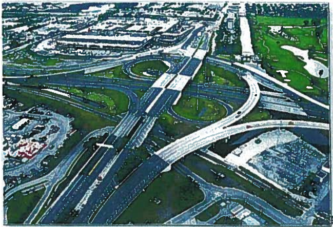
Figure B.2.1-4. Miami Intermodal Connector. This project reconstructed 3 miles of roadway in front of the international airport, and included construction of 11 bridges and associated ramps.
